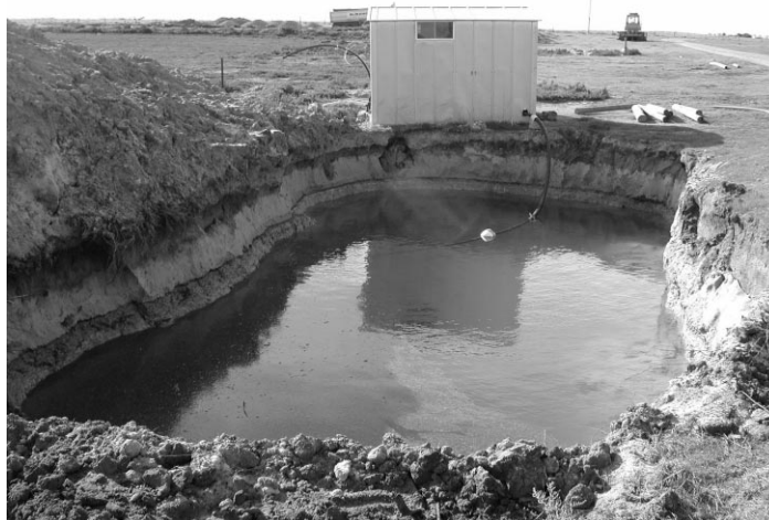
Figure1: Saline groundwater (36-42ppt) is obtained by excavating into the ground at the BGIS, which is pumped to storage tanks for aeration.
