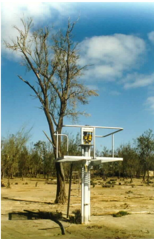
Photograph 4. An air displacement pump on the floor of Toolibin Lake.
